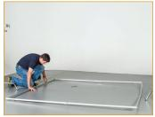
Fasten the latches over the hinges in the middle of all four sides to lock the 8 foot sections in place.
